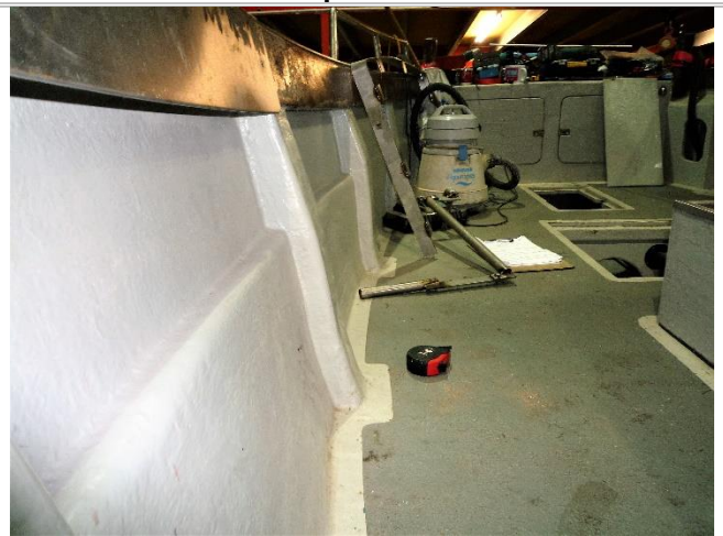
Looking aft stbd. side & run of frames. The frame measurement given is the minimum size as seen here
